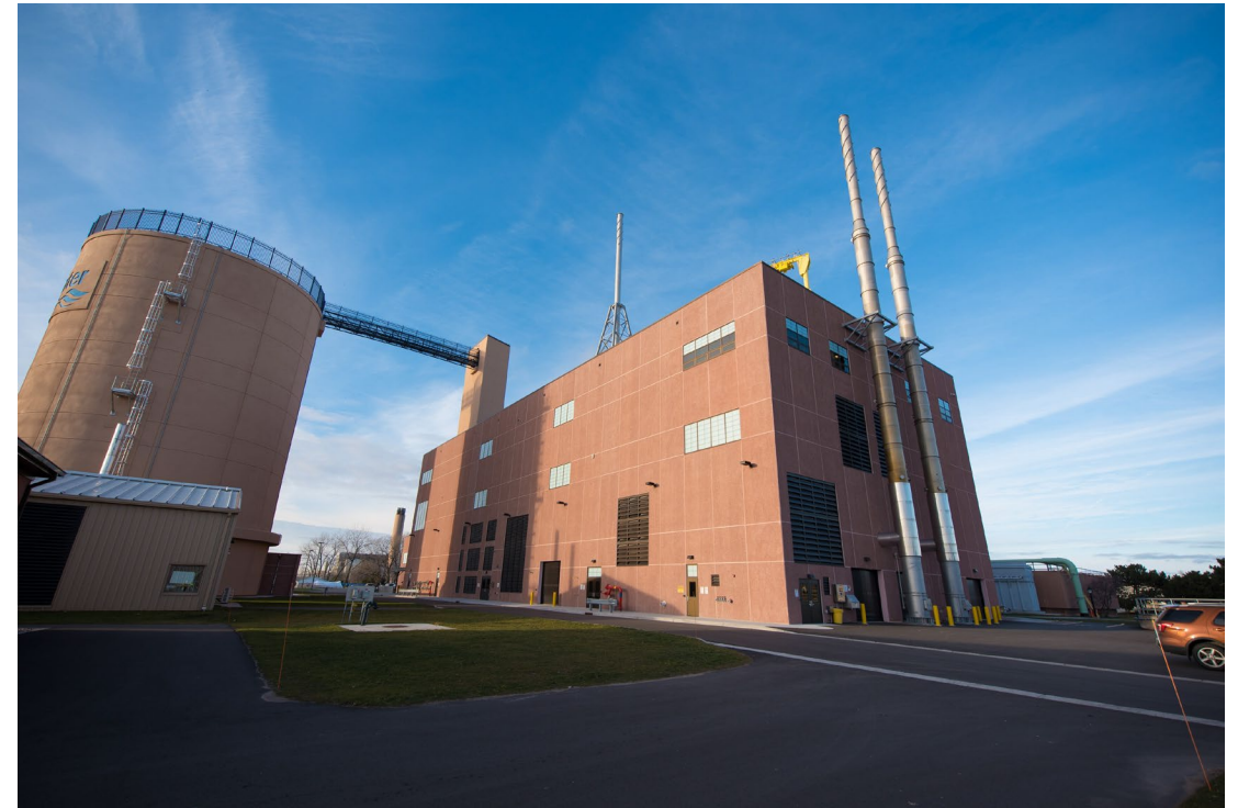
NEW Water in Green Bay, WI transformed its biosolids process with the R2E2 Project, combining anaerobic digestion and fluid bed incineration
