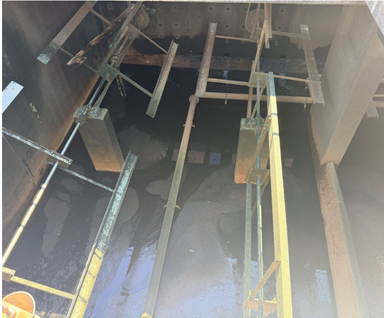
Equipment repair and upgrades – mixing equipment, flocculators, plate settlers, sludge collectors (chains and flights)
