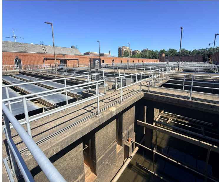
Structural repairs of concrete tankage
