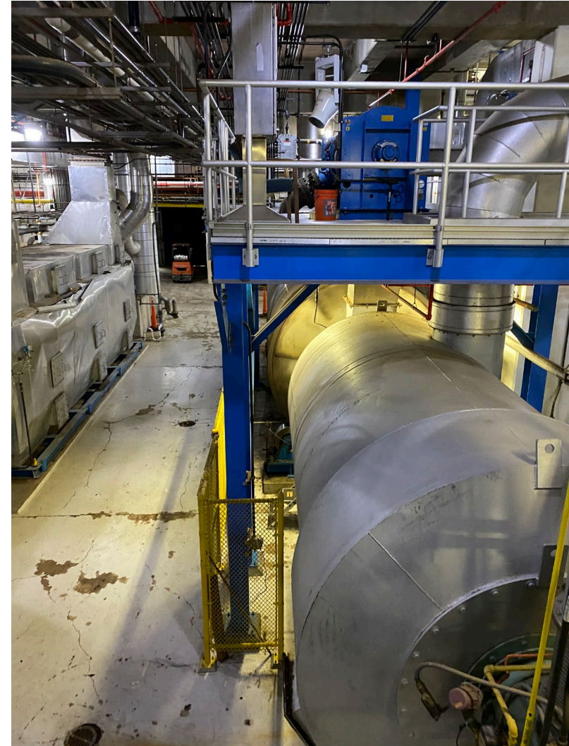
Upper Occoquan Service Authority biosolids thermal drying facility
