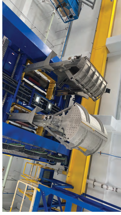
Screen rake and clamshell installed in the screening room
