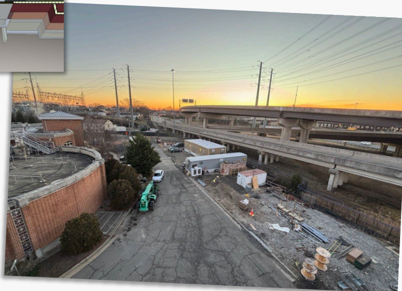
PhaseForward's construction office complex was established
