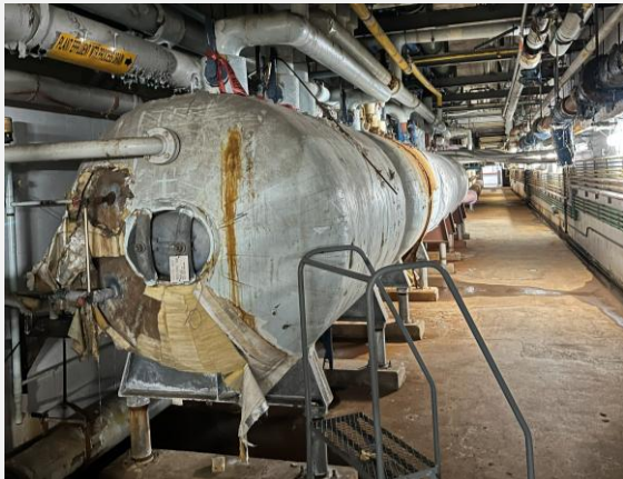
Repair four (4) condensate surge tanks
