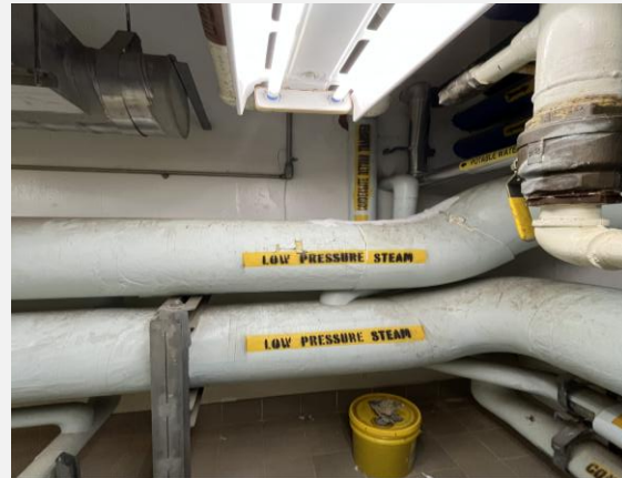
Replace 500 linear feet of steam piping throughout the galleries
