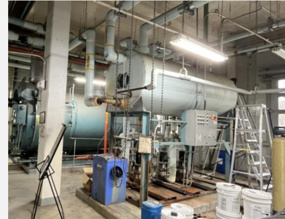
Replace existing boiler feed unit, pumps, and control systems in Building 28
