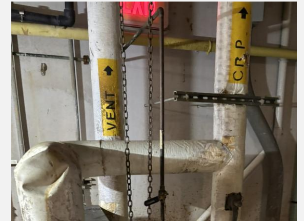
Replace 2,100 linear feet of condensate return piping.
