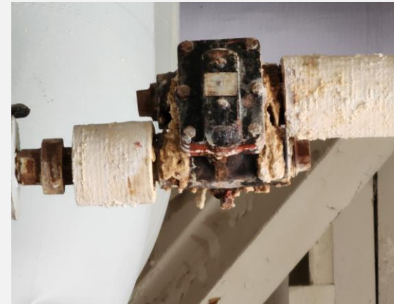
Replace 75 steam traps and valves on the condensate return and transfer pipes
