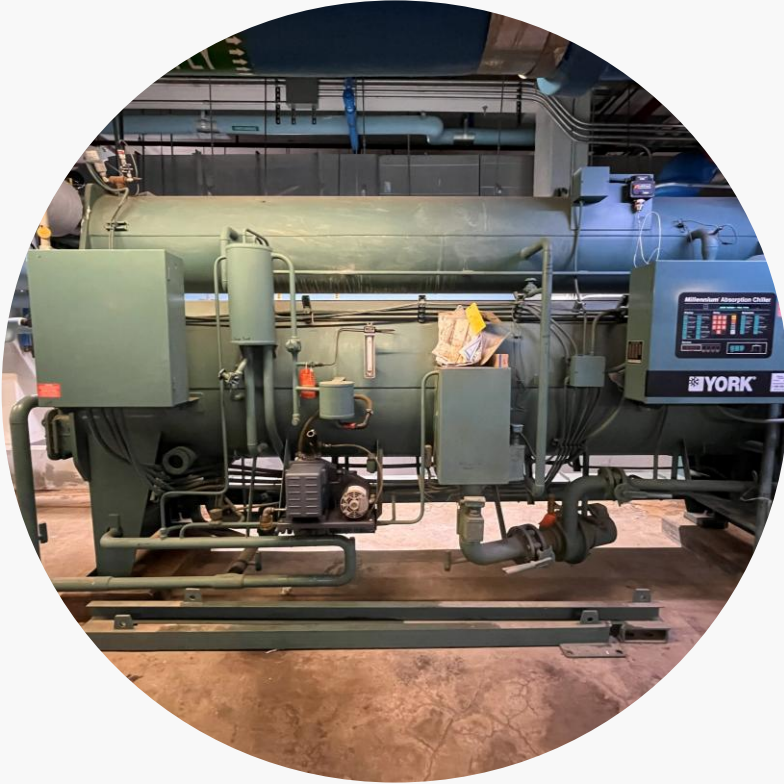
Absorption Chillers. Steam is used as part of the refrigerant process to provide air conditioning.
