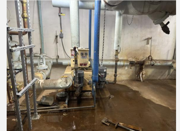
Replace 25 condensate return units and their control panels
