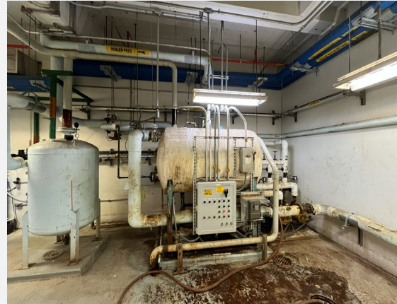
Replace existing boiler feed unit, pumps, and control systems in Building A
