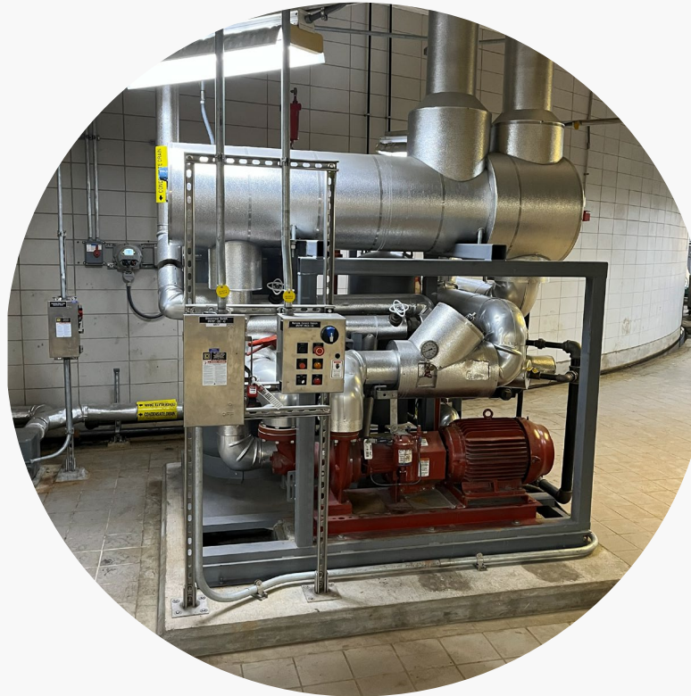
Anaerobic Digestion. Steam is supplied to a heat transfer package to heat water for pasteurizing sludge ahead of land application.
