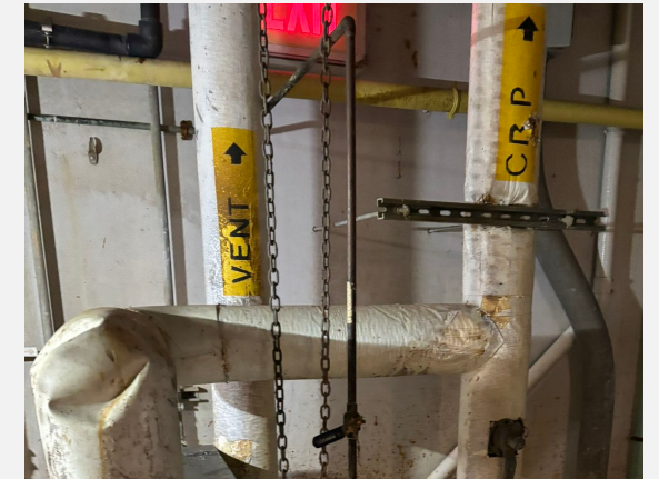
Replace 2,100 linear feet of condensate return piping.
