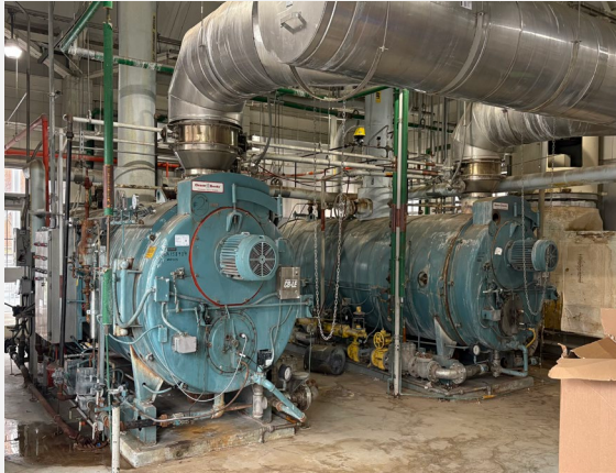
Replace one (1) existing boiler including chemical feed, piping, and control systems in Building A
