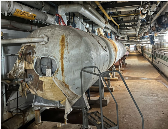
Repair four (4) condensate surge tanks
