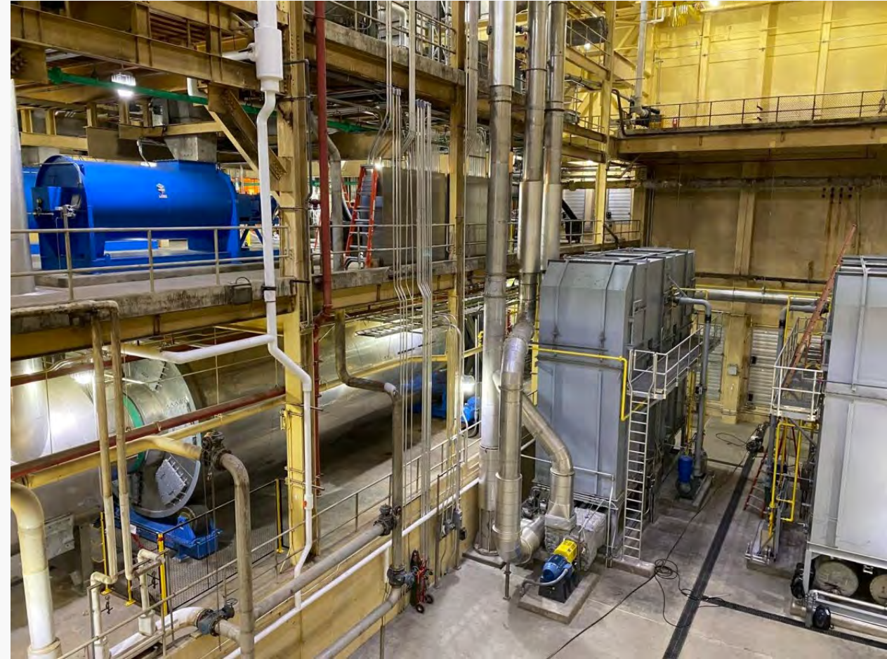
Louisville, KY thermal drying system for biosolids
