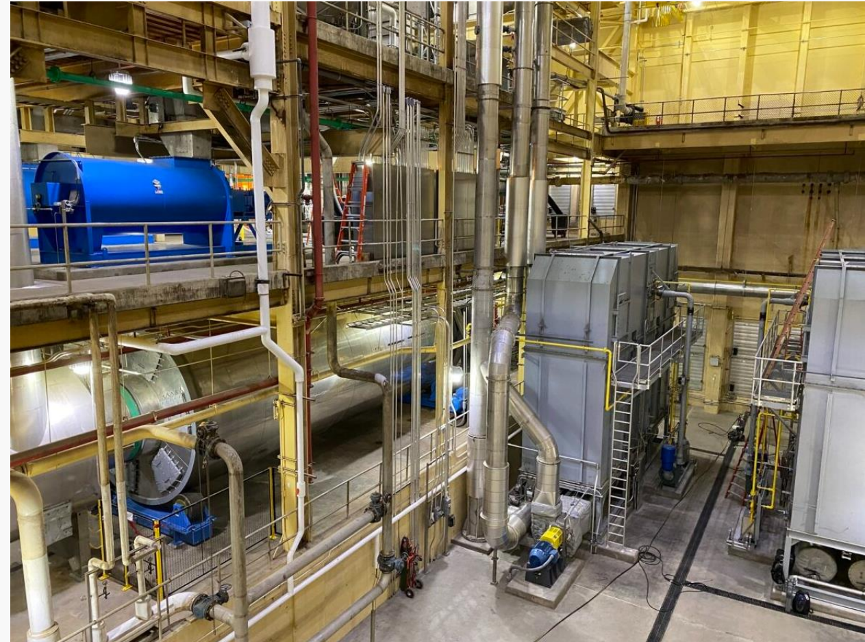
Louisville, KY thermal drying system for biosolids
