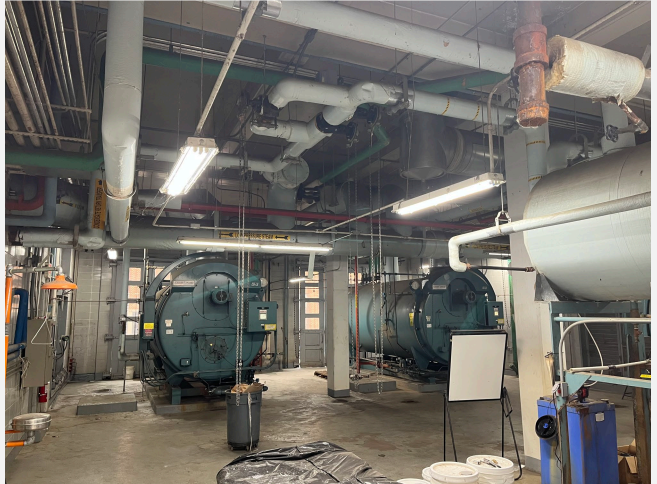
AlexRenew's Natural Gas Boilers in Building 28
