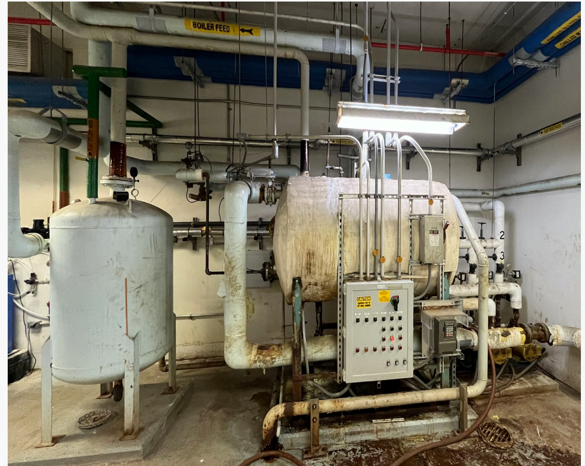
AlexRenew's Boiler Feed Water Unit
