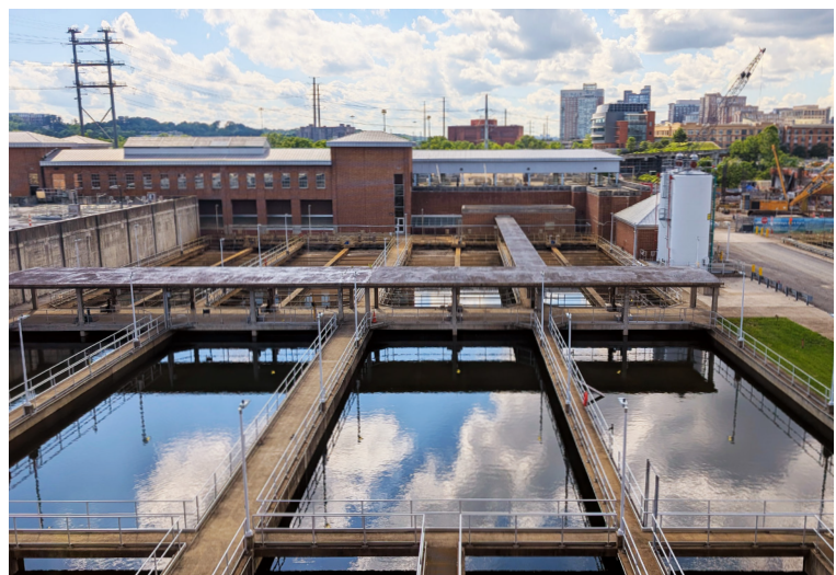
AlexRenew's secondary settling tanks and Biological Reactor Basin.
