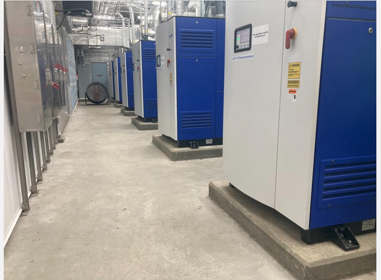
AlexRenew's Process Air Compressors
