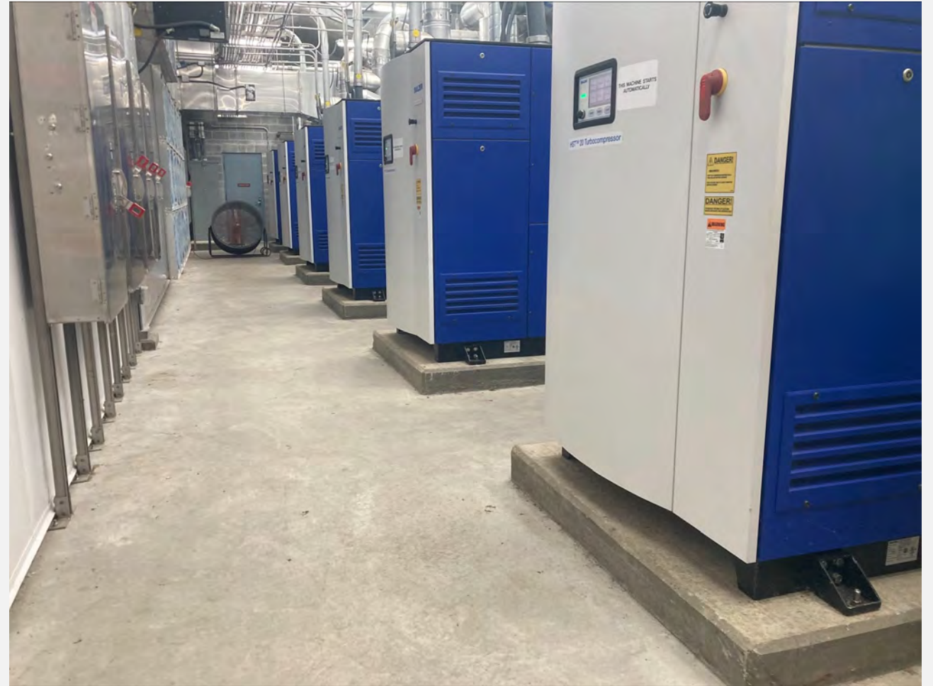
AlexRenew's Process Air Compressors
