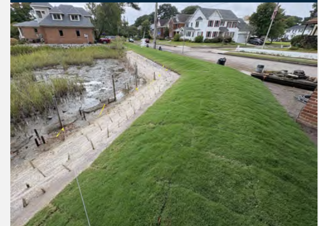
Perimeter Flood Berm/Wall
