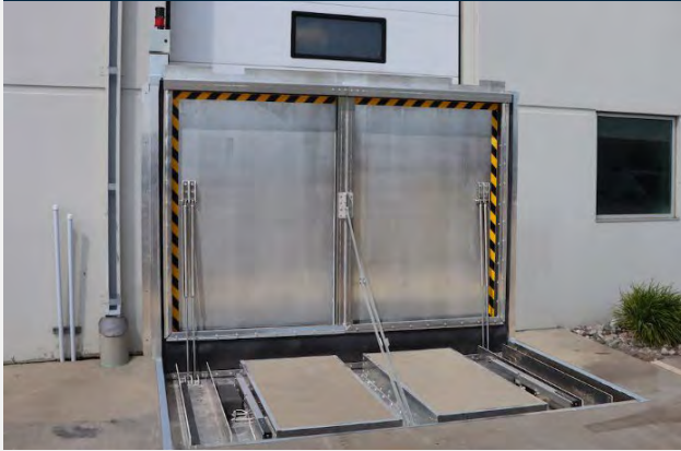
Automatic Flood Barrier
