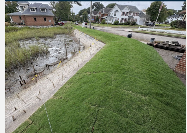
Perimeter Flood Berm/Wall
