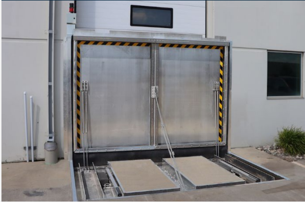
Automatic Flood Barrier
