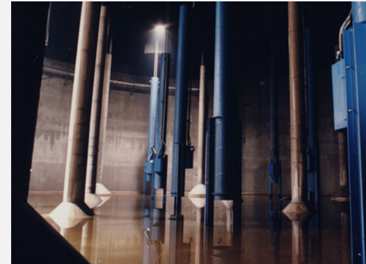
Decommission and demolish the existing gas mixing system and replace with hydraulic jet mixing
