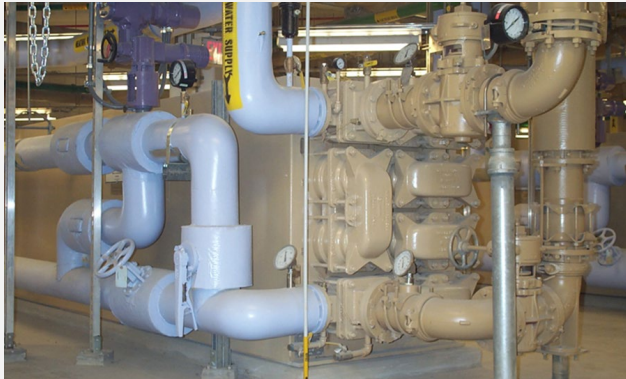
Replace digester heat exchangers (4) with larger units to provide all digester heating
