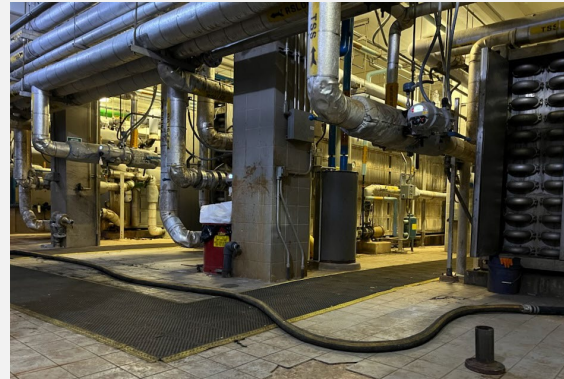
Decommission and demolish the pre-pasteurization system include heat exchangers (3), solids pumps (6), and storage tanks (4)
