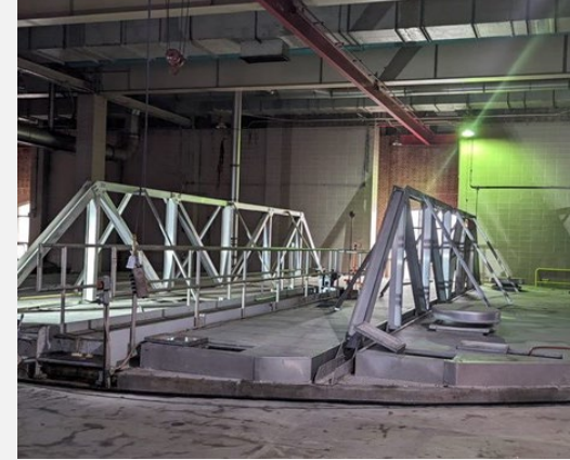
Full refurbishment of gravity thickeners (3) with new rake drives, piping, scum collection systems, covers, and controls
