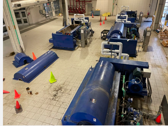
Replace existing thickening centrifuges (4) and add fifth dewatering centrifuge along with obsolete drive motors
