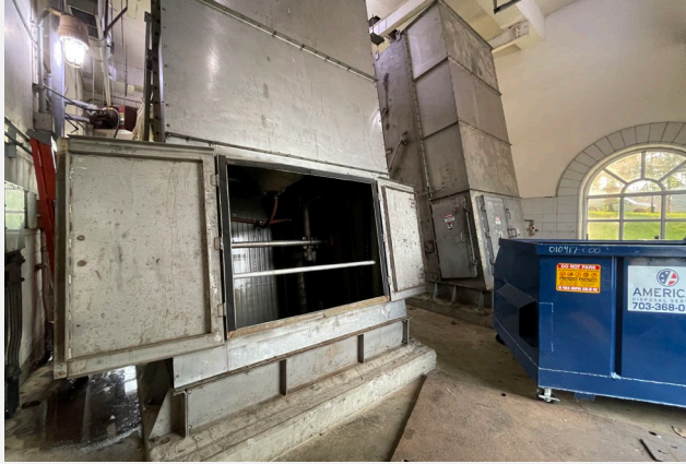
Upgrade existing coarse screens (2) and add third coarse screen channel and equipment
