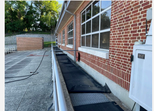
Repair concrete and install new covers over the primary effluent channel
