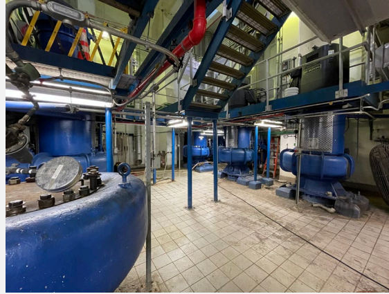
Replace existing Raw Sewage Pumps with new pumps, valves, and piping to a firm capacity of 120 MGD
