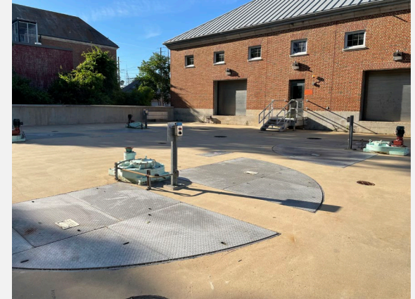
Replace two (2) vortex grit separators and add three (3) stacked tray grit separators
