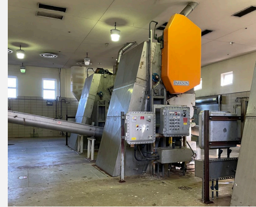
Upgrade existing Fine Screens and conveyers to capture more screenings
