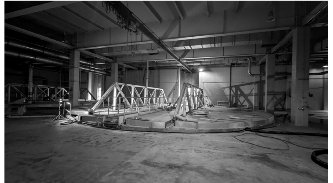
Gravity Thickeners at AlexRenew
