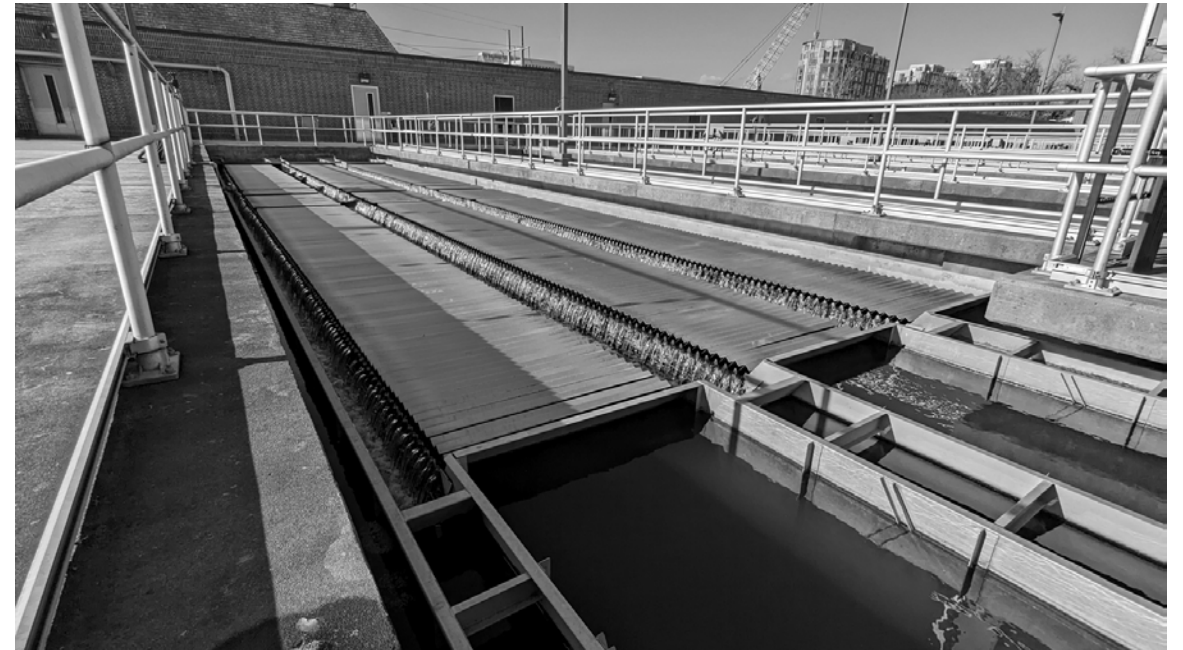
Tertiary Settling Tanks at AlexRenew
