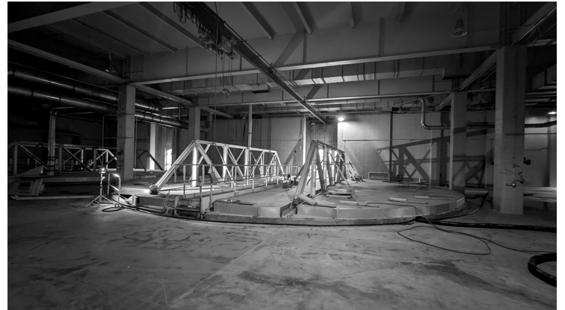
Gravity Thickeners at AlexRenew
