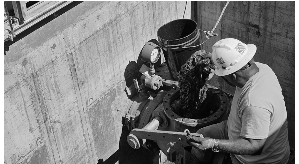
Valve replacement at AlexRenew
