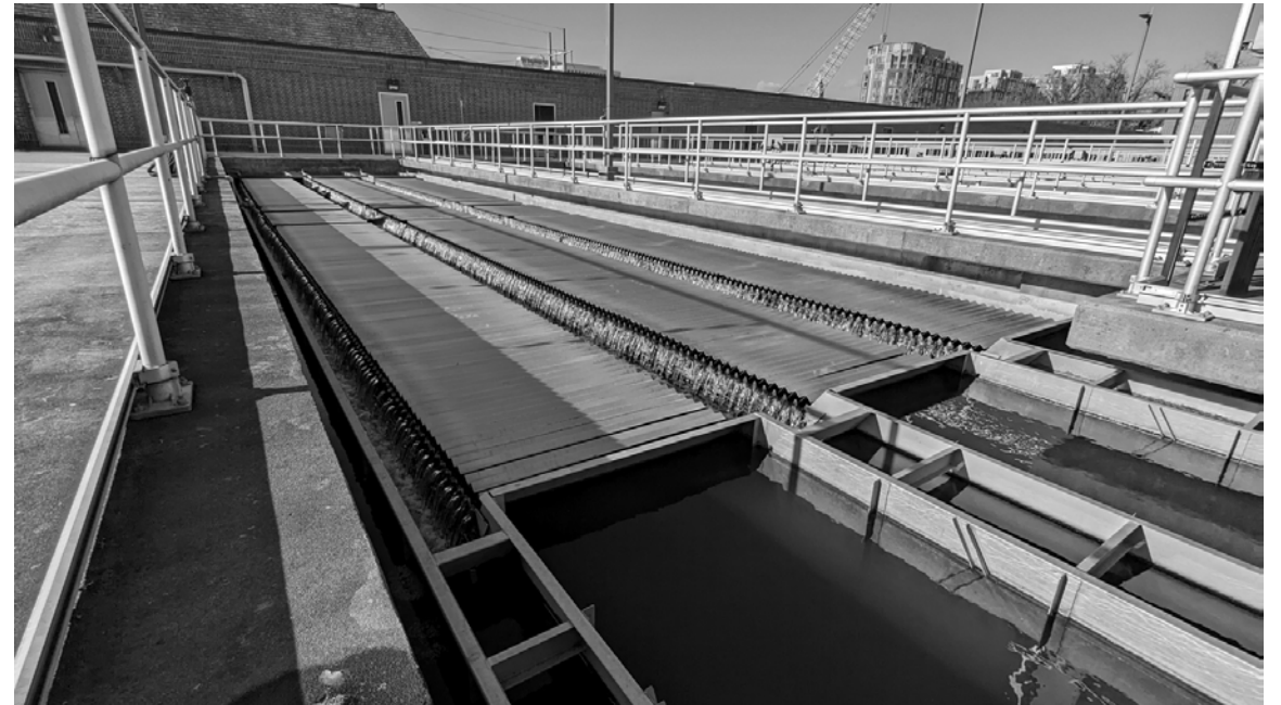
Tertiary Settling Tanks at AlexRenew
