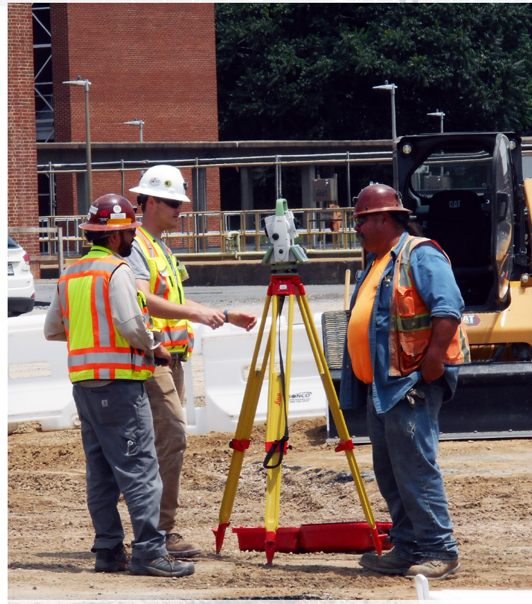
Crews conducting survey work in Alexandria
