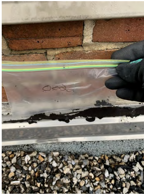
Photo 3 - Sample 002 black/silver sealant on metal flashing
