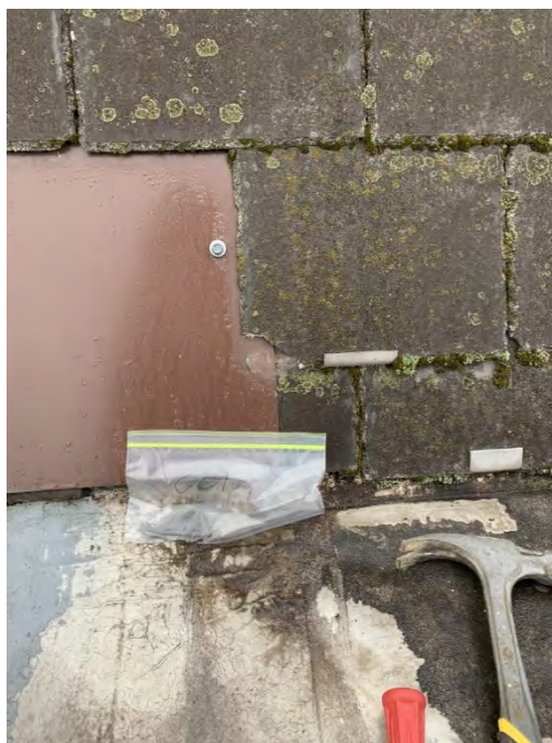
Photo 1 - Sample 001 fibrous cement tile 10% Chrysotile ACM
