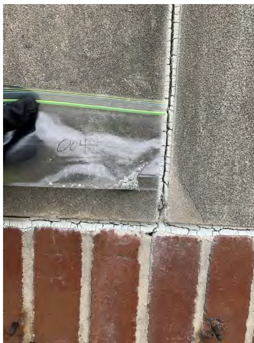
Photo 7 - Sample 004 white caulking in stonework joints
